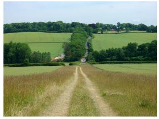
top of the hill. The quality of the original construction is still apparent, with the road being somewhat raised above the adjoining fields and having a drainage ditch on either side. Three kilometres (two miles) behind the photographer, the Roman road passes beside a Roman burial mound that today is only about a metre high. It marks the most southerly point of Elmdon parish - where it meets both Clavering and Langley.
